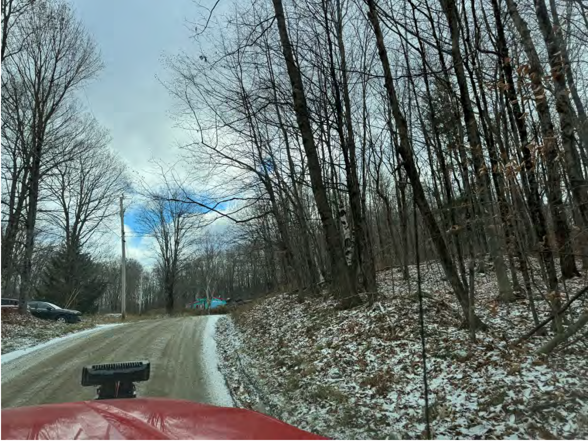
28900 before 7 – finish stone line ditching on right at top of hill
