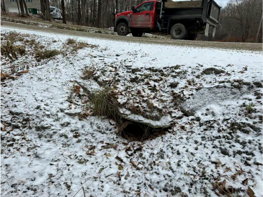
28900 before 4 – Culvert 1 replacement with 24" pipe
